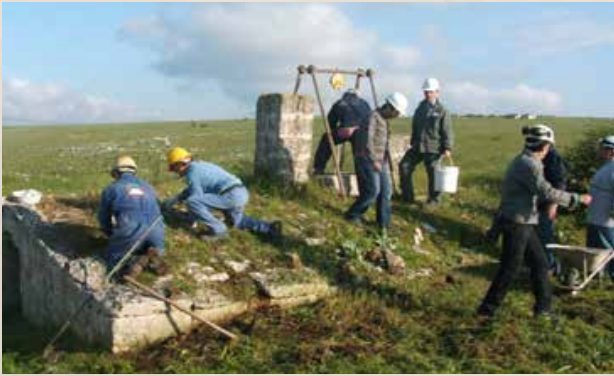
Training and restoration of cisterns.
