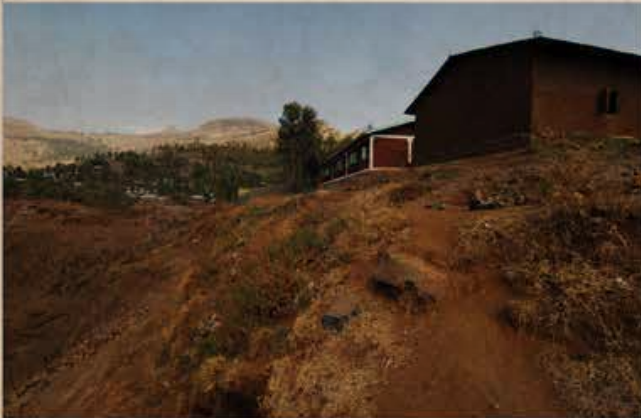
The hillside in front of the school, before the restoration work.
