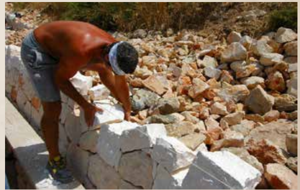
Training and restoration of the terraced slopes.
