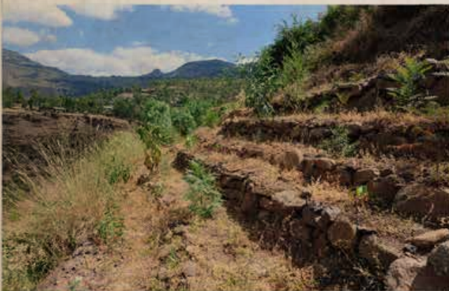
The hillside in front of the school, after the restoration work.
