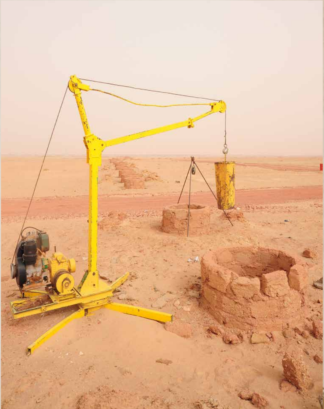
Works in progress in Adrar, Algeria.
